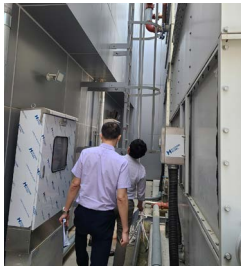
Inspection of cooling tower
